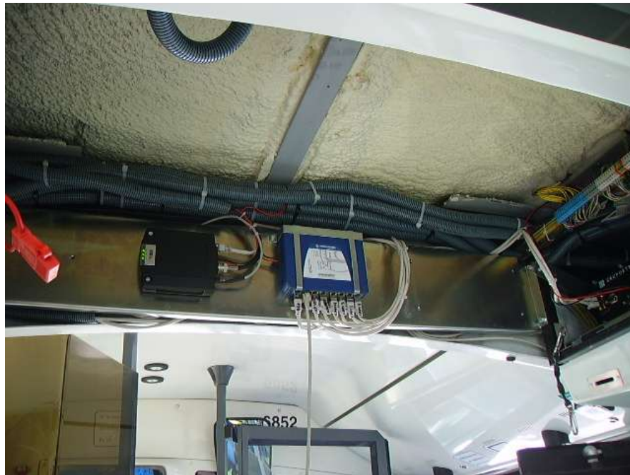
Figura 2 – Frontal del armario principal
